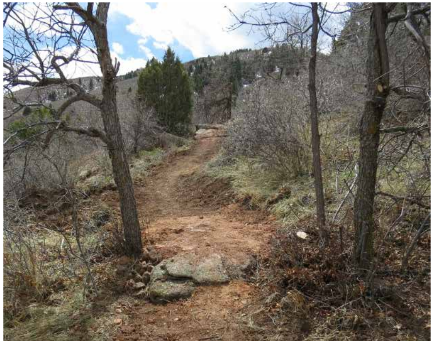
Example reworked trail with hardened water bar with outflow for runoff.
